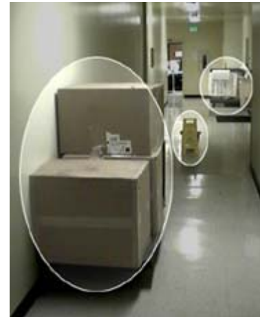
Obstacles in hallways may prevent passageways from providing the required width to accommodate a safe evacuation.
